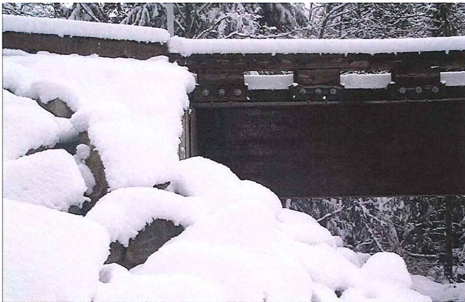
CK2443 Side View Abutment Left Bank
