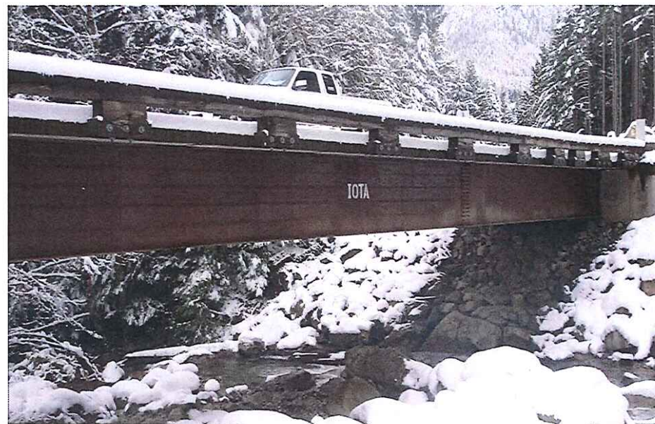
CK2443 Crossing Upstream
