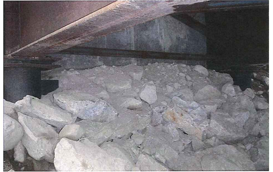
CK2443 Abutment Left Bank
