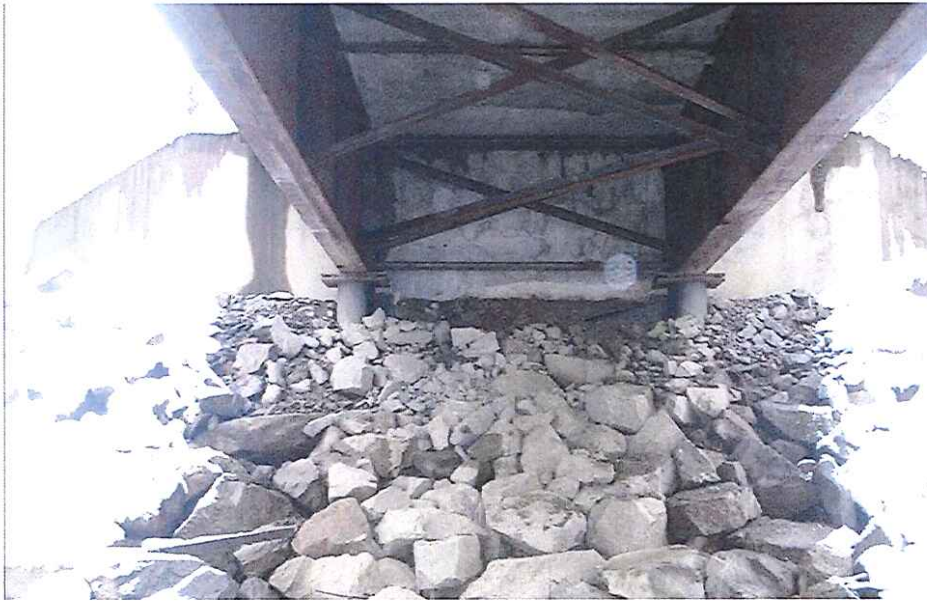
CK2443 Abutment Right Bank
