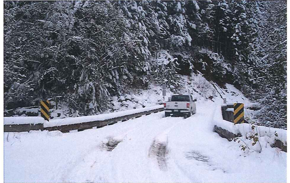
CK2443 Approach Right Bank
