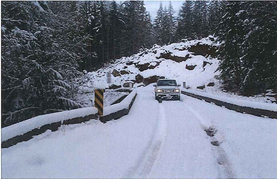
CK2443 Approach Left Bank
